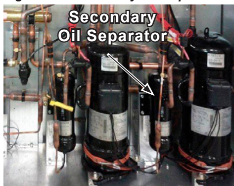
Figure 16: Secondary Oil Separator
