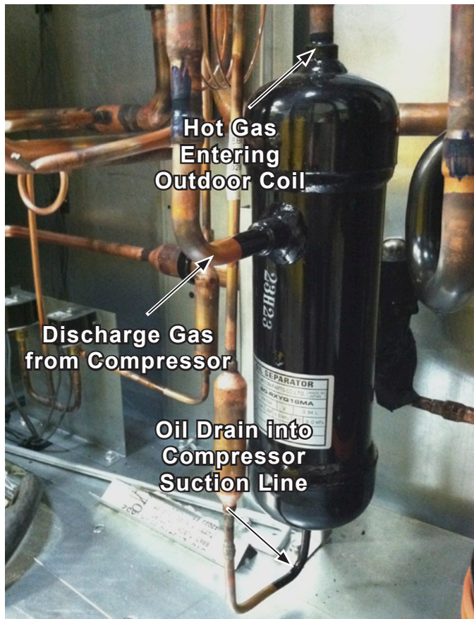
Figure 16: Secondary Oil Separator
