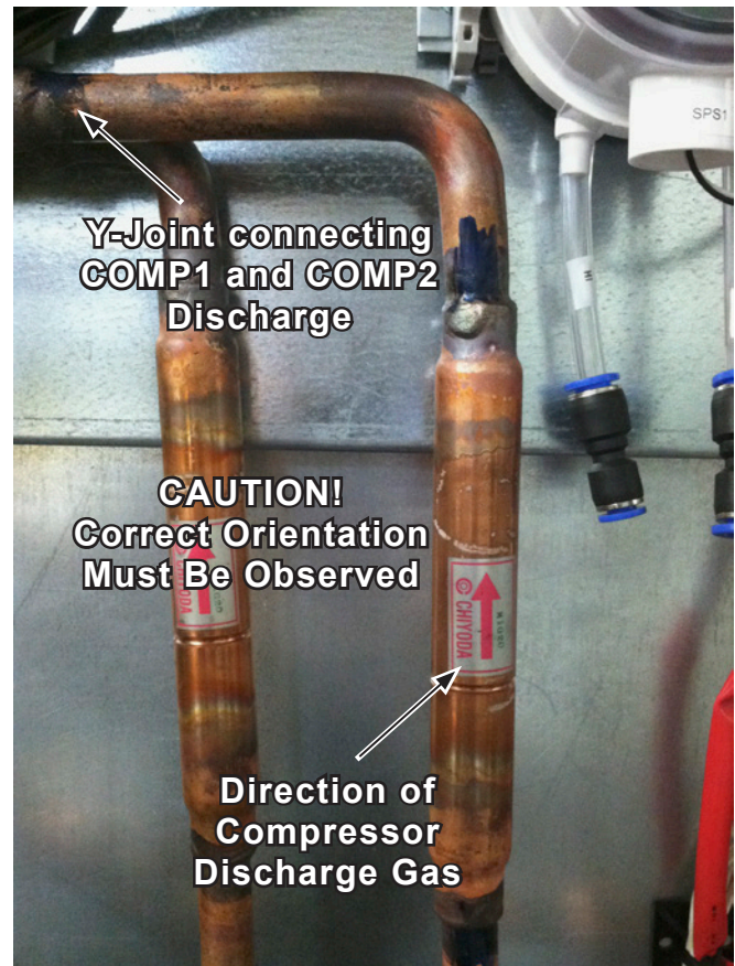
Figure 17: Discharge Line Check Valves on Large Cabinet (7.5T) Heat Pump (DPH)
