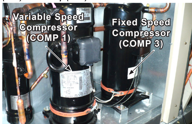
Figure 13: Compressor Tandem on Large Cabinet (7.5T) Heat Pump (DPH)
